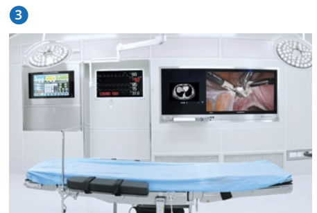
Shanghai No. 10 People's Hospital Shanghai, China
